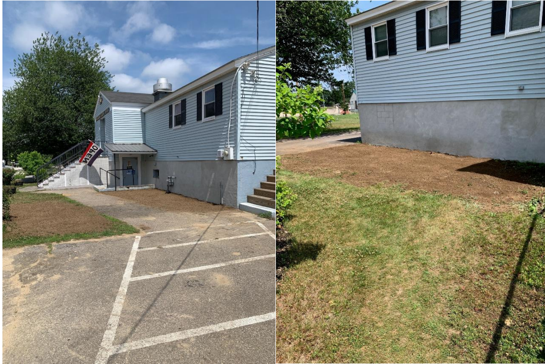
Front of building stucco work.
