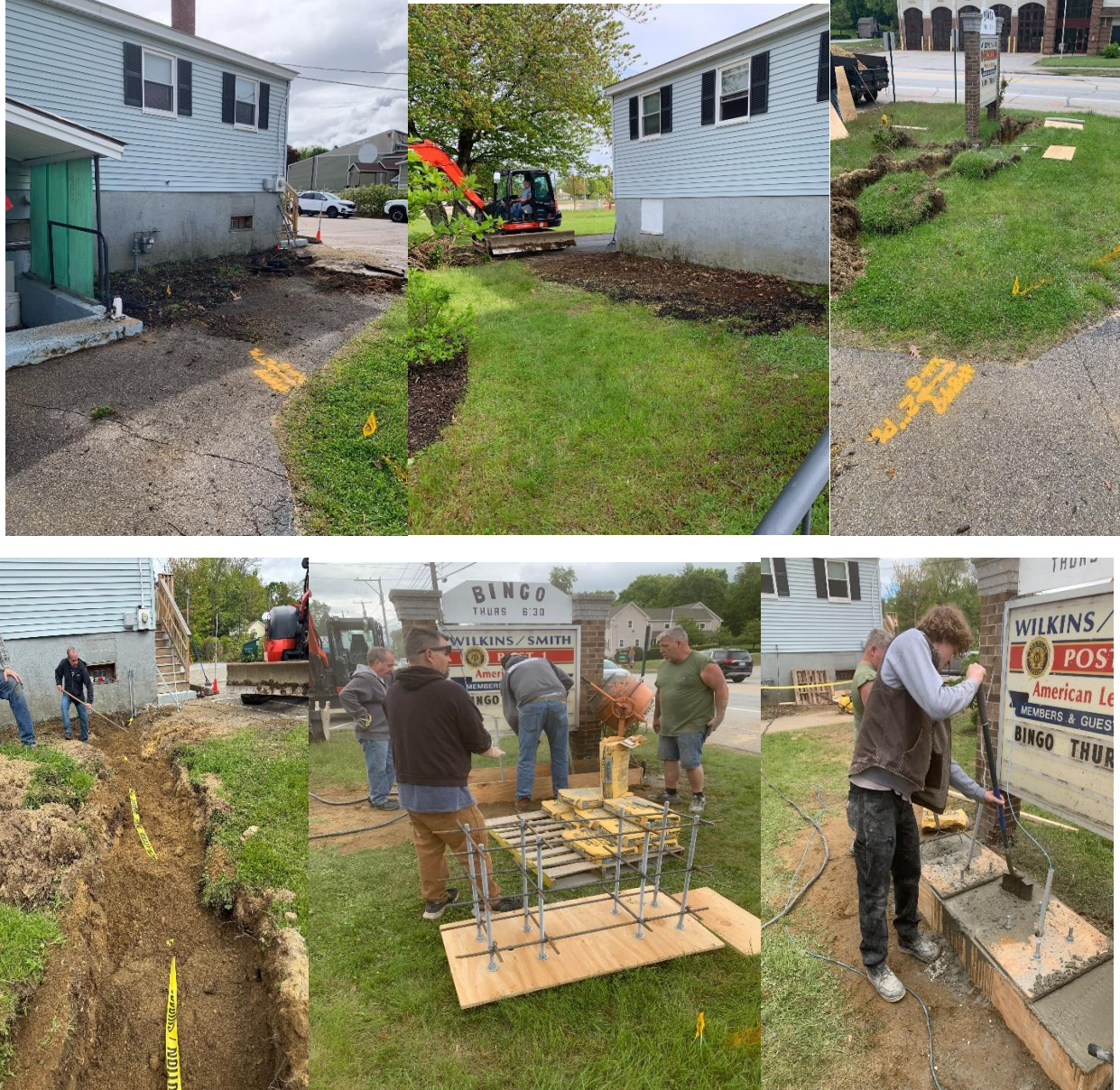
Removing the hedges, digging a trench, placing new conduit, and a new footing and finally pouring concrete! Thanks to all the volunteers that made it happen!
